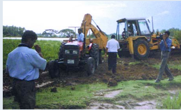
Restoration work at 'Uduwila Wewa'
