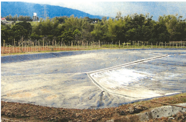
Biogas Plant in Rocky Farms, Pililia, Rizal.
