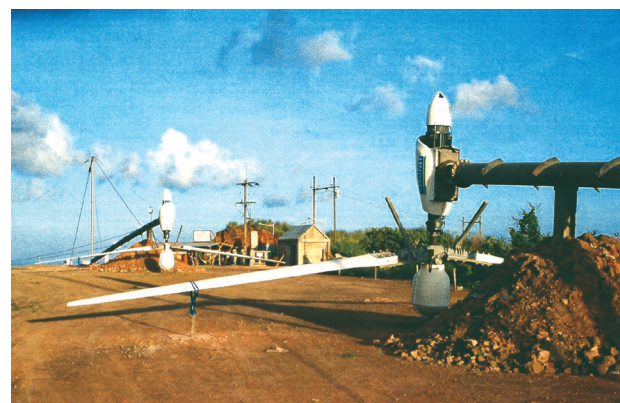
Hybrid Wind-Diesel System Project in Makatao, Batanes, in its installation stage.
