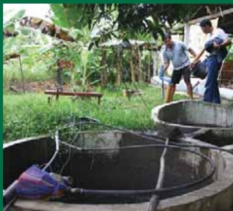
Bio-gas project of Cebu CFI. One of the notable projects of consistent Gawad PITAK winner and Hall of Famer Cebu CFI is its Bio-Gas which processes and converts gas from animal manure to provide an alternative, cheaper and odorless source of fuel energy ideal for home use.
