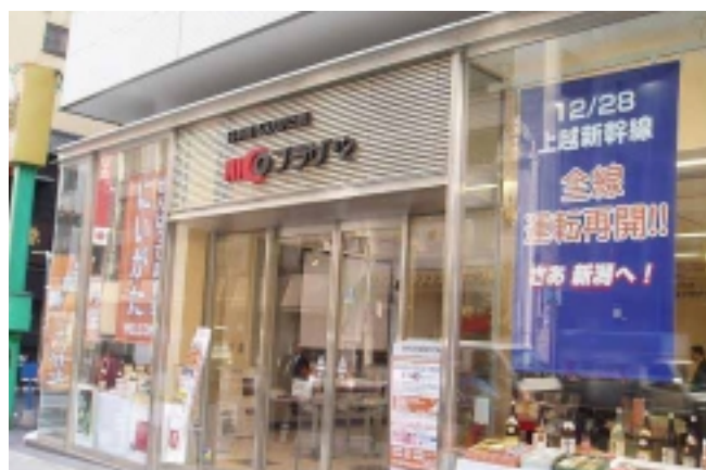
The 1 st and 2 nd floors of the Tokyo Branch building are being provided to the Niigata Prefectural Government's Industrial Creation Organization (NICO), and are used by many of Niigata's enterprises.
