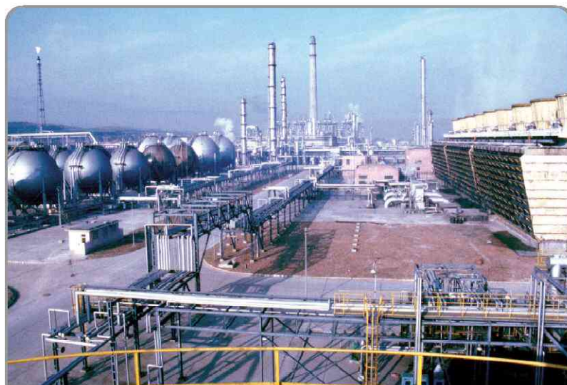
Project of Shandong Qilu Petrochemical Company Supported by the Bank
